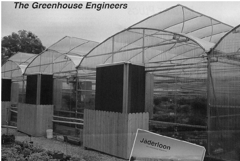
Steel Pipe Arch polycarbonate glazing
